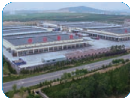
WEIHAI HAIDU 60000T LOGISTICS COLD STORAGE PROJECT
