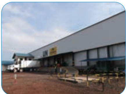
UNITED NATIONS LOGISTICS COLD STORAGE PROJECT IN CONGO KINSHASA
